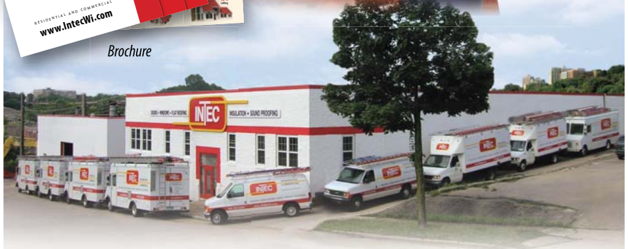
Building Identification and Fleet Vehicle Lettering
